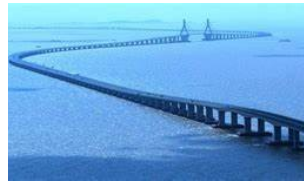
Donghai Bridge - China
