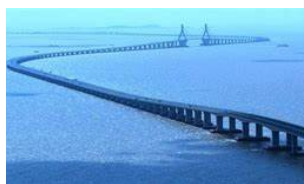
Donghai Bridge - China
